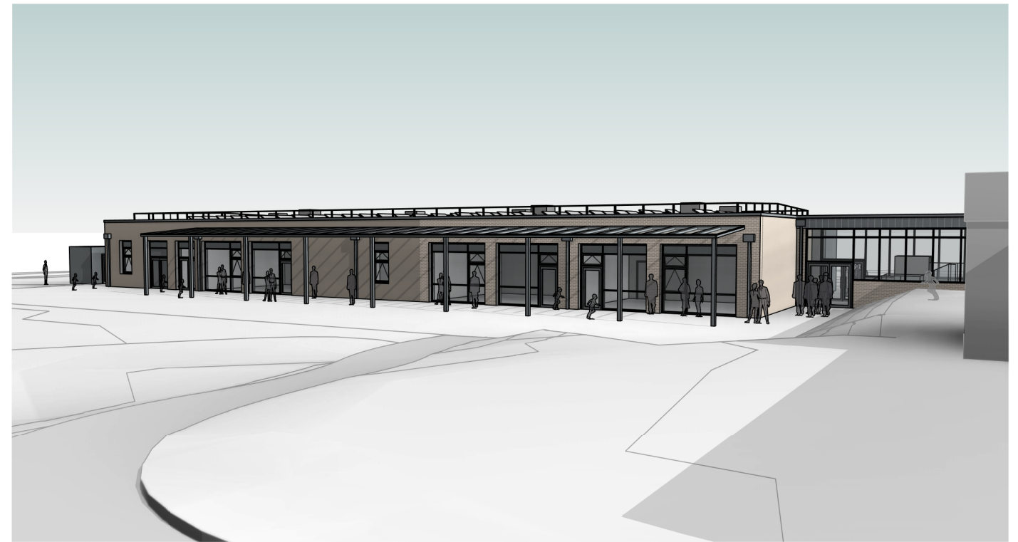
View from the West
